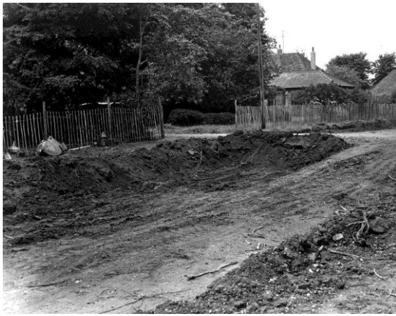
THE EXCAVATION SITE NOW LONGSTAFF WAY
